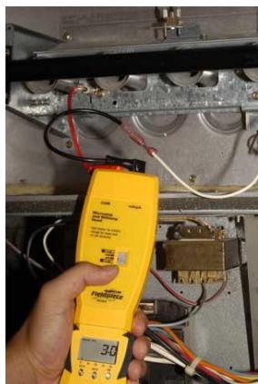
**0 microamps:** Look for an open or grounded sensor wire or flame rod, or a defective module. The wire and rod can be diagnosed with an ohmmeter. Check the flame sensor. Make your diagnosis of a defective module after all other possibilities have been checked.
