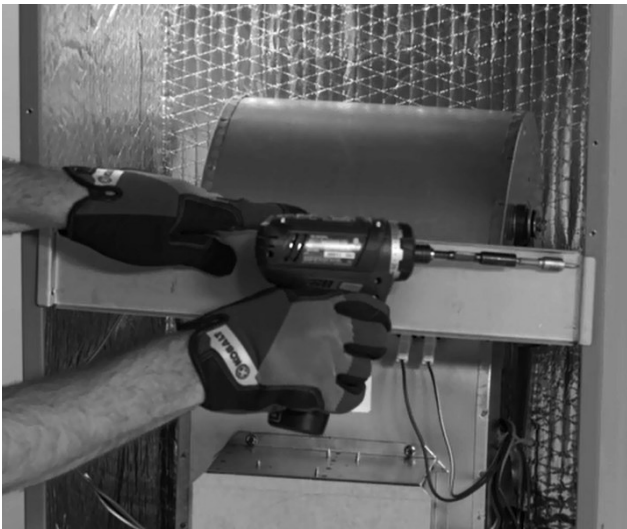
Installing Support Bar
