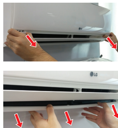
Figure 21: Removing the Bottom Cover (Appearances Will Vary Depending on Indoor Unit Model).
